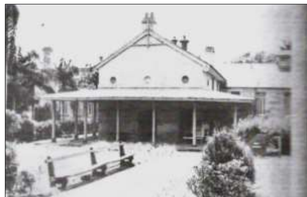
Parramatta Psychiatric Centre, records storage room 1975.
